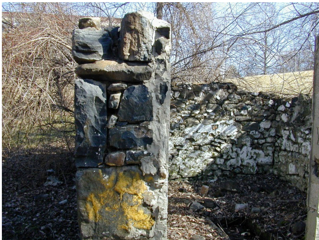
Remnants of the Pratt springhouse
